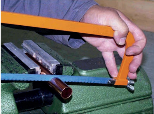
1. Rectangularly saw off the pipes
